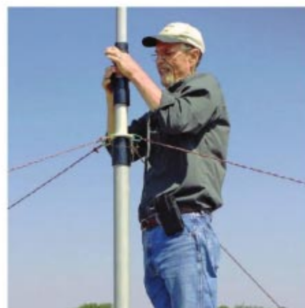
Figure 6 — Dayle Good, KK6HNS, pushing up mast sections while helpers gently hold the top guy wires.
